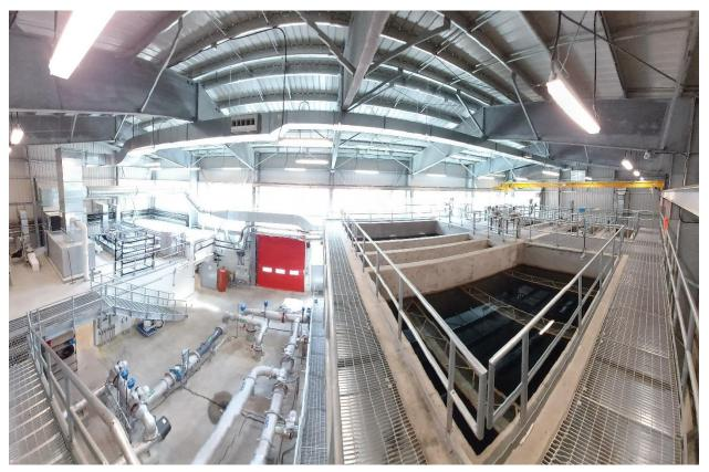
Interior panoramic showing (from right to left) the HVAC system, pipe gallery with UV disinfection system, anthracite/sand media filters, flocculation tanks.
